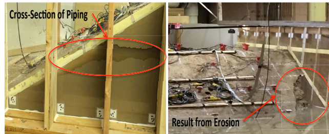
Fig. 3: Experimental earth embankment built at the USBR showing cross-section result of a piping induced by the removal of the rebar (left) and result of significant erosion of materials from piping (right).
